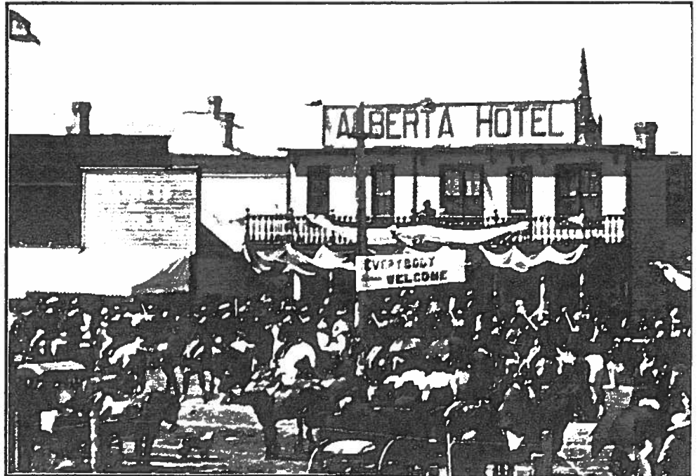
Fig. 1 Claresholm Main Street former Railway Avenue now Highway #2, July 1, 1906
