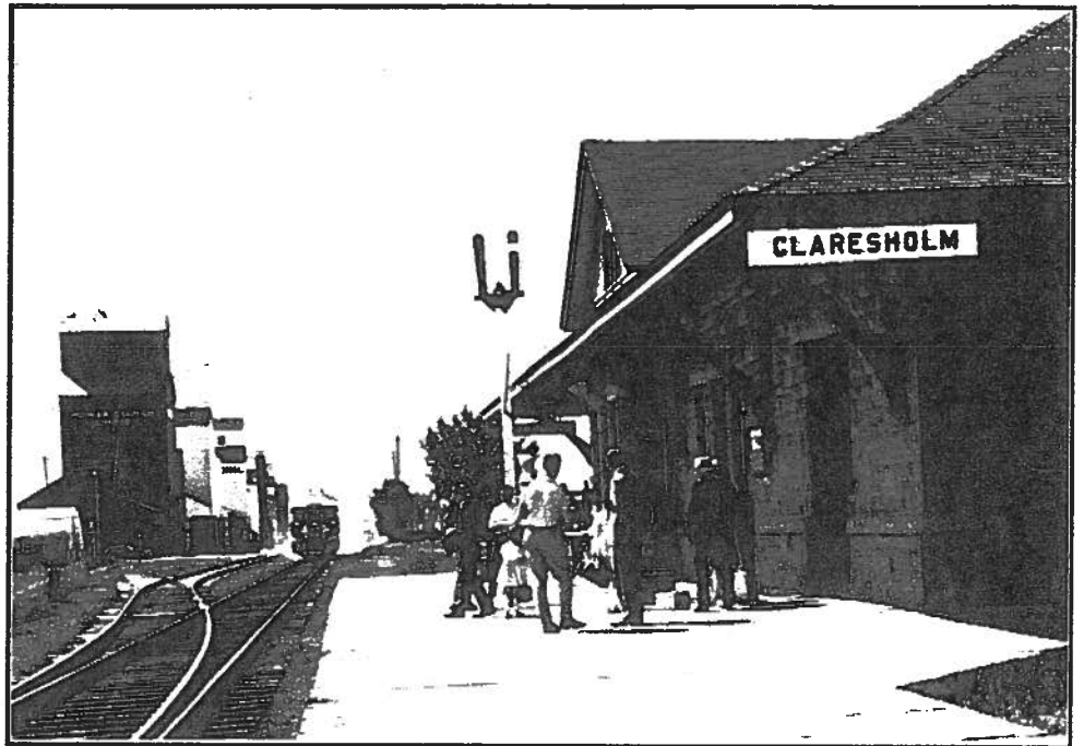
Fig. 4 Claresholm CPR Train Station was constructed in 1912 of sandstone quarried from the first Calgary CPR station
